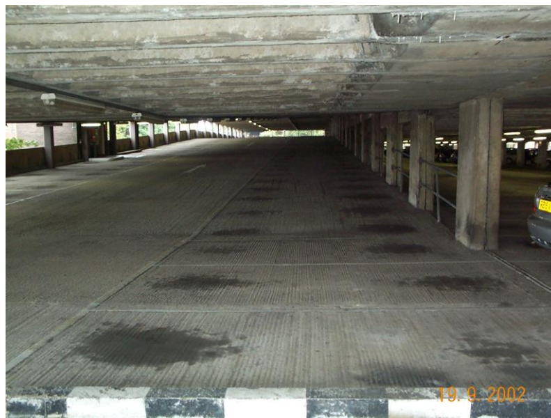
Figure 3: View of Car Park before rehabilitation program began
