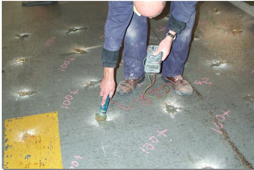
Figure 6: Half-cell testing of parking decks
