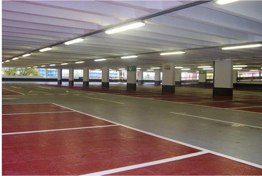
Figure 8: Enhancement of social aspects through better lighting and colour-coding of parking and pedestrian features gives the parking structure added sustainability credentials
