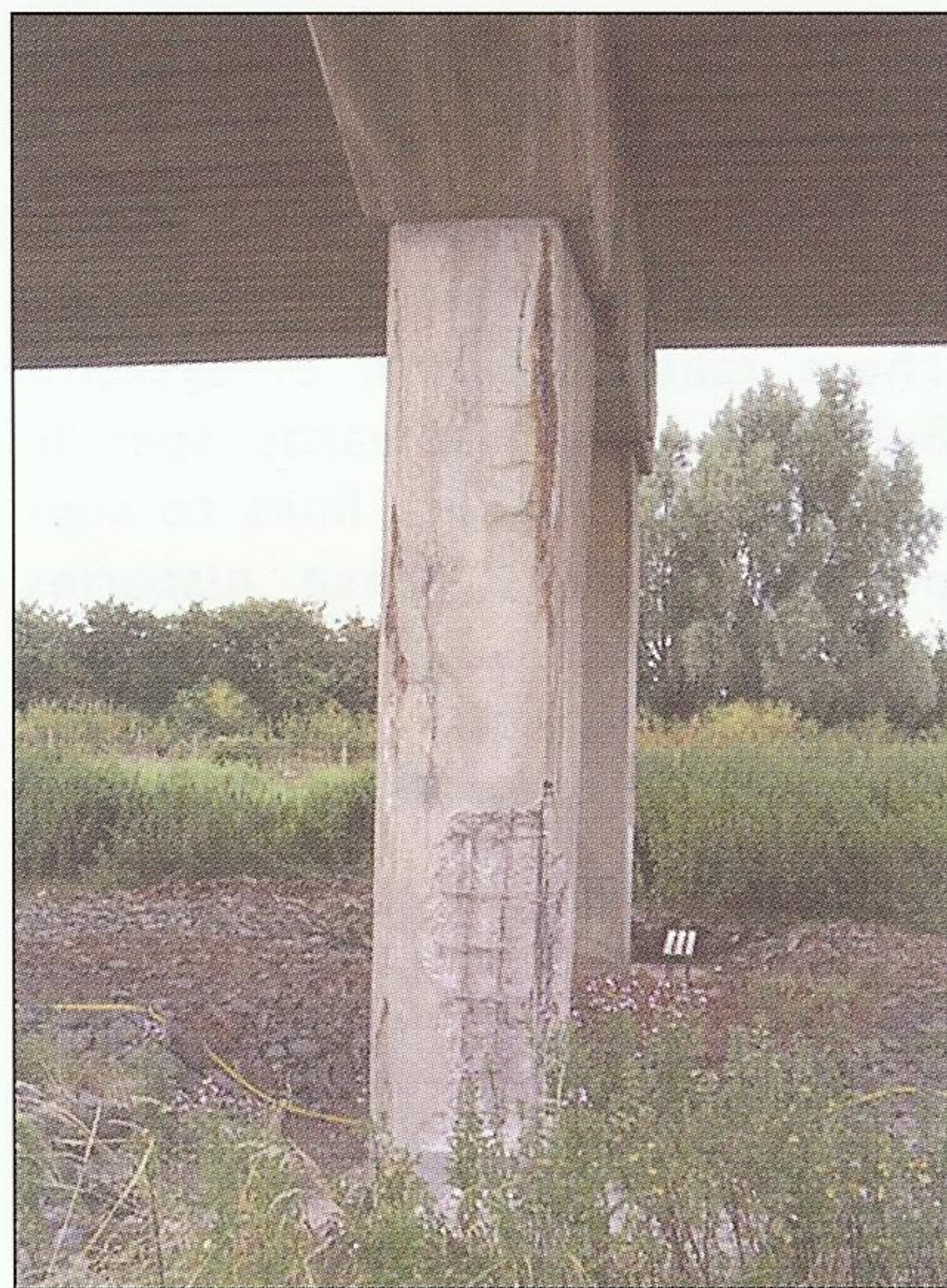
Highway bridge undergoing extensive repair due to corrosion.
