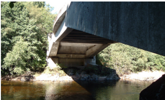
Historic Reinforced Concrete Bridges in Aberdeenshire were repaired and beams and half-joints protected in 2005 (Dinnet—above) and 2008 (Bervie Jubilee—below) and are managed in an integrated AiMS site for the County Council.
