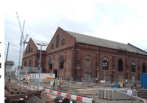
DIMCO Buildings (right) were built in the 1920s as the first inner city power station in Europe. Refurbishment was completed in 2007 with ICCP installed they are now powering the White City shopping complex in London.
