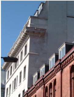
Phoenix House (left) is a thriving office building in the centre of Manchester that has benefited from discrete anode ICCP installed to all elevations to 8 levels in 2003.
