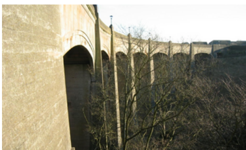
Historic Reinforced Concrete Bridges in Aberdeenshire were repaired and beams and half-joints protected in 2005 (Dinnet—above) and 2008 (Bervie Jubilee—below) and are managed in an integrated AiMS site for the County Council.
