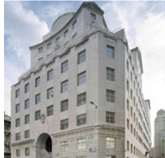
Phoenix House (left) is a thriving office building in the centre of Manchester that has benefited from discrete anode ICCP installed to all elevations to 8 levels in 2003.
