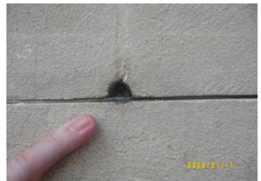
Discrete ICCP anodes and monitoring devices were installed within the bed joints intersecting stone blocks and small "Dutchman" repairs to maintain an aesthetic finish.
