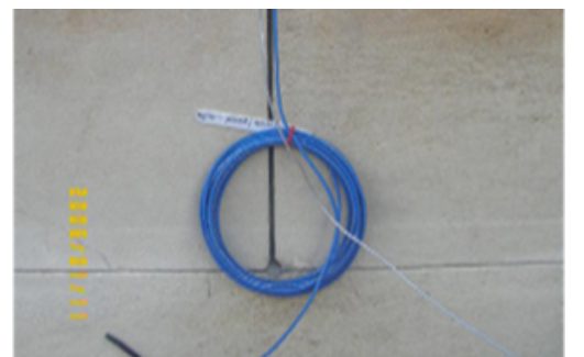
Discrete ICCP anodes and monitoring devices were installed within the bed joints intersecting stone blocks and small "Dutchman" repairs to maintain an aesthetic finish.
